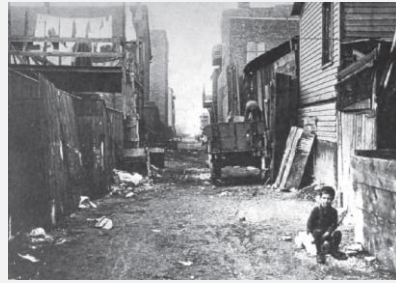
Photo 1.4: The general insanitary conditions which surround the houses on both sides of the alley. The first house on the right is a small dilapidated frame house. Beyond it are three larger tenements. The outbuildings at the left are all dilapidated, and contain privies which are in a foul condition. There are not enough garbage boxes to supply the needs, and the ones provided are so seldom cleaned that the families dump their slops and garbage in the alley. (1901)
